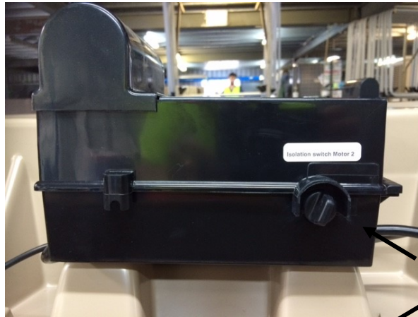
Motor No. 2 Iso- lation Switch
