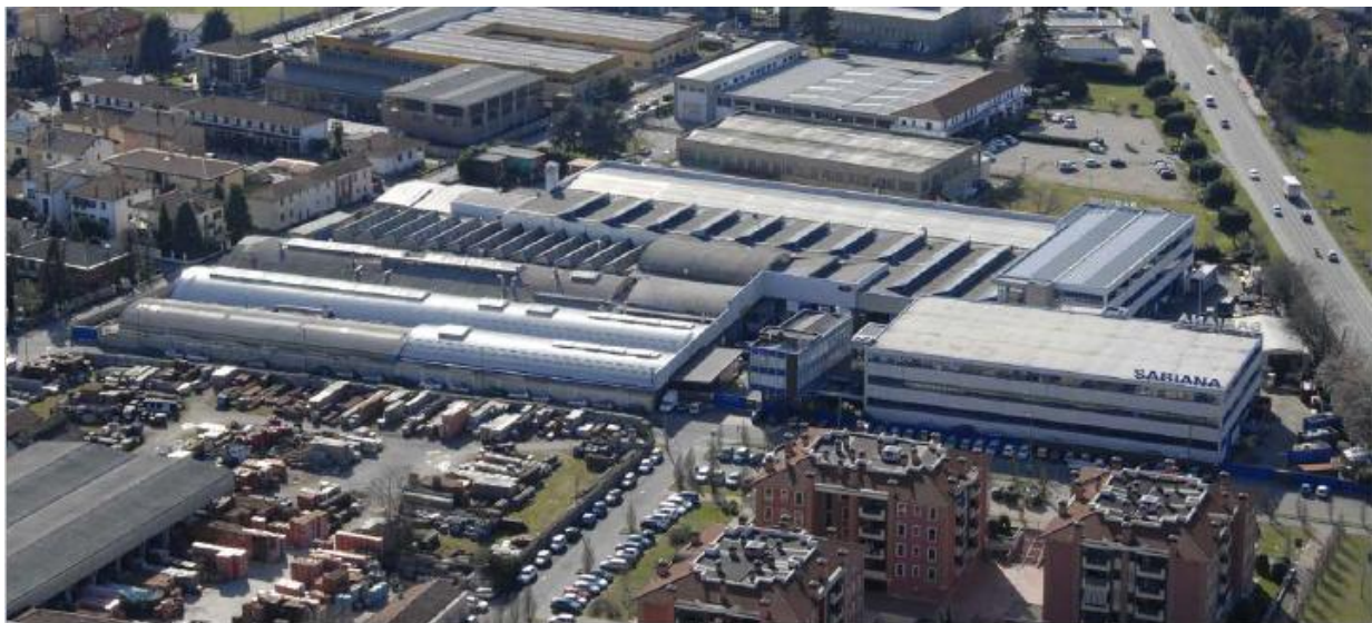
Aerial view of Sabiana headquarter
